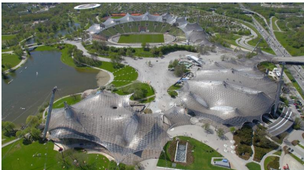
Fig.9 Acrylic panels clad the tensile membrane in Munich Olympic stadium [20].
