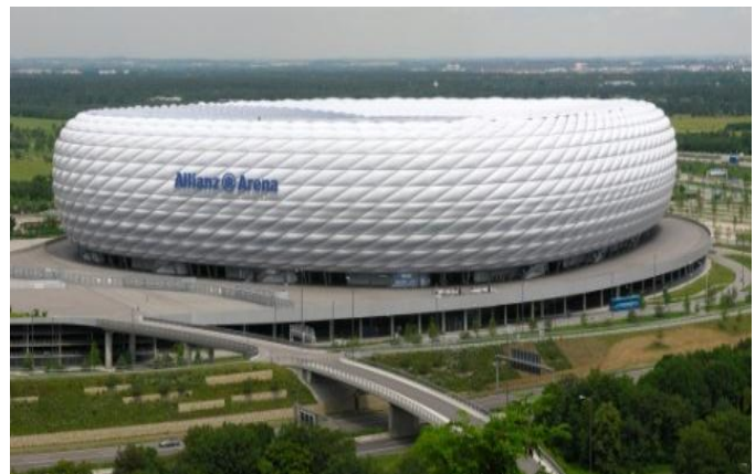
Figure 11: Allianz-Arena Stadium in Germany looks like a monolithic air - filled ETFE cushions floating above the ground [21].
