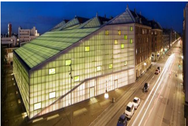
Fig.6 Polycarbonate used as a glazing material in Sports and culture center in Holmbladsgade, Copenhagen [16].
