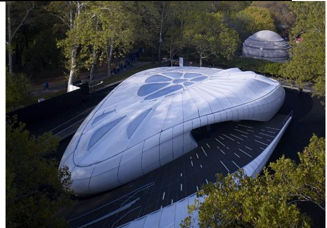
Fig.5 GRP (glass fiber reinforced polyester) was chosen as an ideal cladding material for Chanel mobile art pavilion in central park, New York [10].
