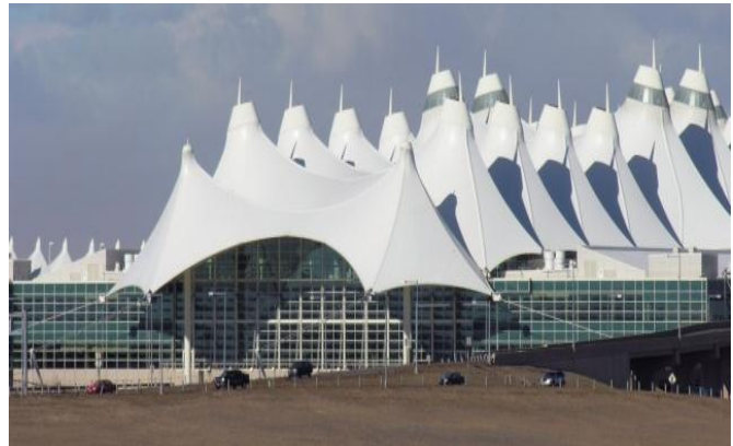
Fig.10 The roof of Denver International Airport consists of a series of PTFE tent-like modules [24].
