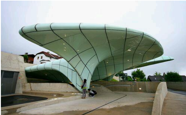
Fig.8 Glass fiber reinforced polyester was used to clad Nordpark railway station entrance [21].
