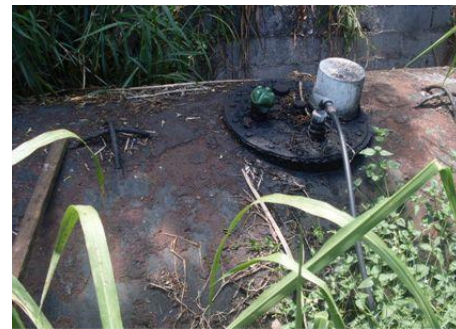
Fig. 6 Corroded digester
