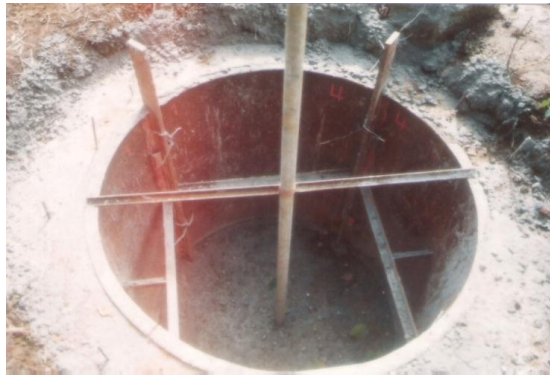
Fig. 3 Support for gas holder
