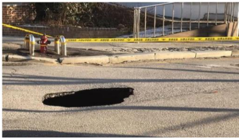
(a) First ground sinking
