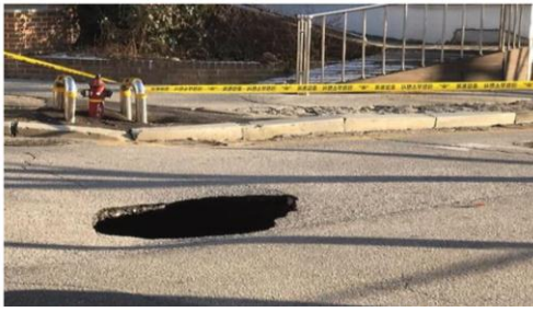
(a) First ground sinking
