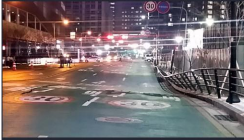
(c) Second road crack and settlement
