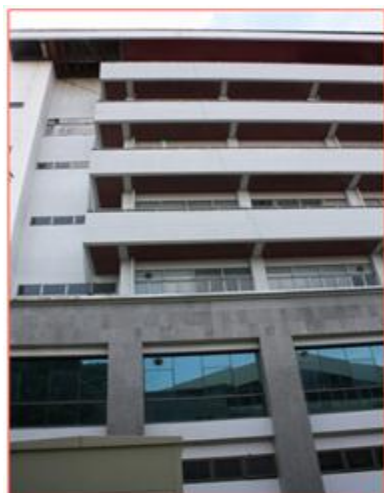
Fig. 3 Civil Engineering Building
