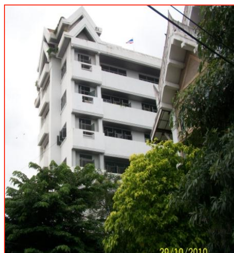
Fig. 2 Phitsanulok City Hall
