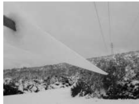
Fig. 1 Ice load on ETL conductor
