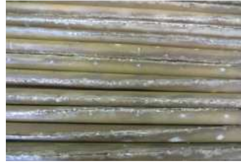
Fig.7. Lateral Distributors Condition
