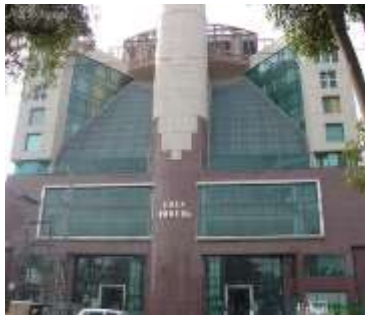
Fig. 6 Eden Tower's Front Façade
