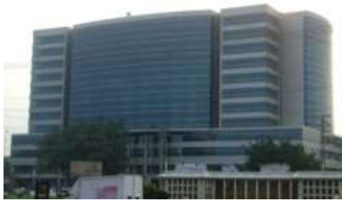
Fig. 7 Front façade of Big City Tower
