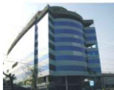
Fig. 3 Mega Tower's Front Façade
