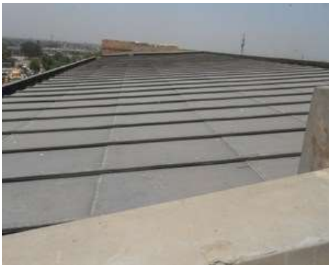
Figure 7: Roof Covered With copper Sheet
