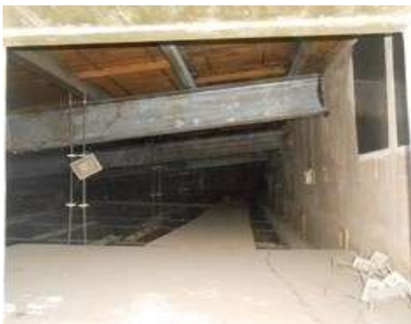
Figure 8: Double Roof with Supporting Hangers
