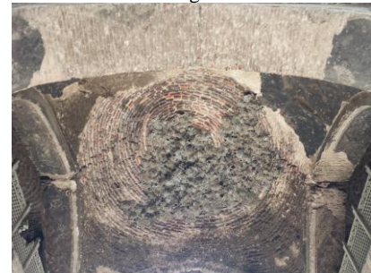
Fig. 11 Scaling seen inside the galib kari
