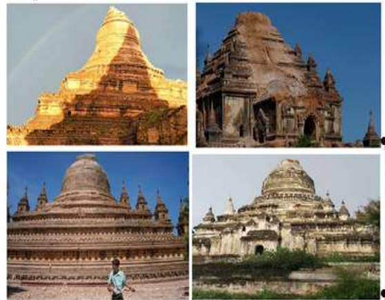
Fig.1 Earthquake damages of heritage structures
