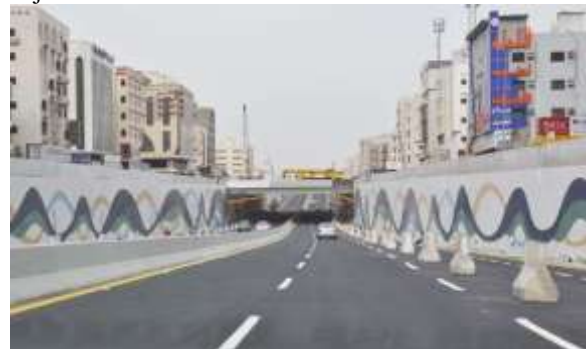
Fig. 4: Travel time from Sitten Bridge to Sabaeen Street now takes just a few minutes with the opening of Tahlia-Makarona underpass in Jeddah Saudi Arabia
