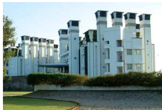
Fig. 3: Passive Downdraft Evaporative Cooling in Torrent Research Centre, Ahmedabad, India
