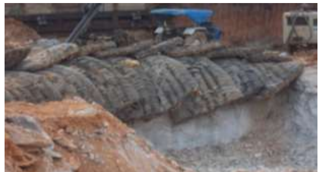
Fig. 3 Muffling Arrangement for controlling Fly Rock
