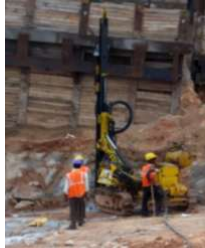
Fig. 2 Drilling of Blastholes in Progress
